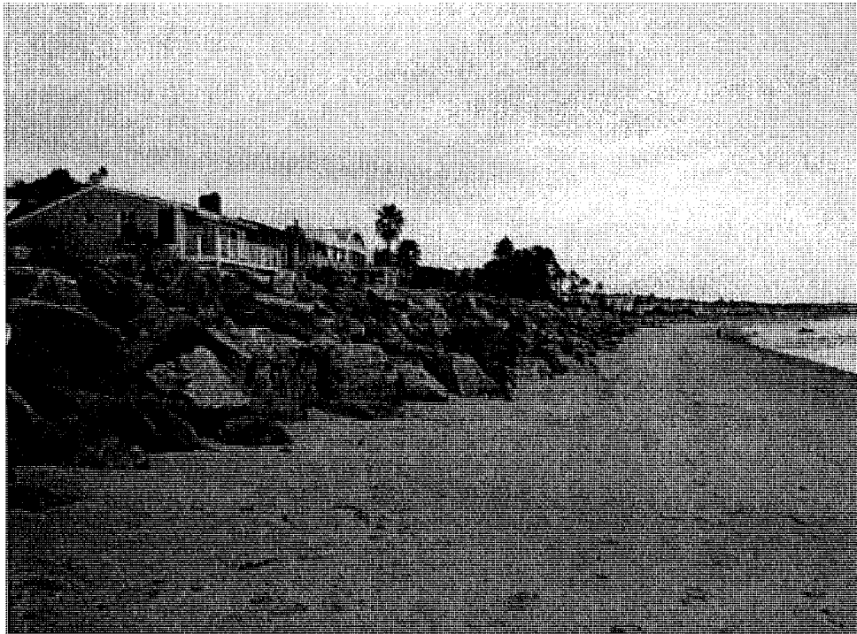
Photo 2-7. Emergency Revetment (February 2010)
