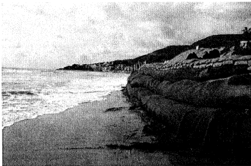
Photo 2-4. Temporary Sandbag Revetment (December 2009)
